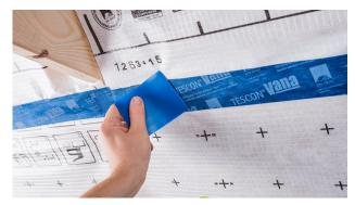
**5b. Rub the adhesive joint firmly** Rub the tape firmly using the pro clima PRESSFIX to secure the adhesive bond. Ensure that there is sufficient resistance pressure.
