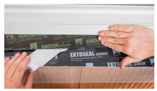
**6. Stick onto the reveal and rub into place** Remove the release film strip and stick the tape all around the window.
