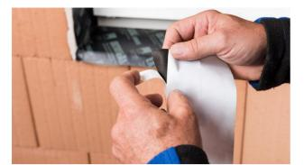
**3. Remove the first release film strip** Remove approx. 5-10 cm (2" - 4") of the narrow release film strip.
