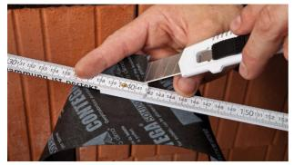
**3. Cut the CONTEGA SOLIDO EXO window-sealing tape** Add approx. 4 cm (1 5/8") to the height of the frame and cut this length of tape.
