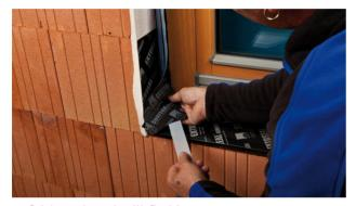
5. Stick to the sub-sill flashing
