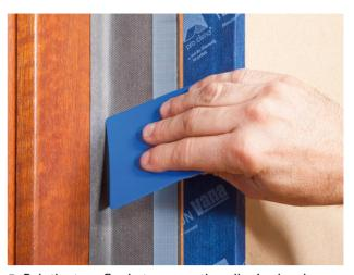
**5.** Rub the tape firmly to secure the adhesive bond Rub firmly using the pro clima PRESSFIX application tool to secure the adhesive bond.
