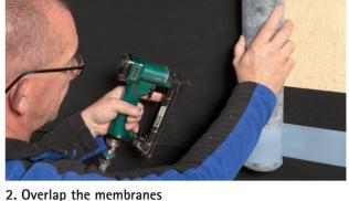
Clean the subsurface (dry and free of dust, silicone and grease). Overlap the membranes by approx. 10 cm (4") so that they are watertight. The printed markings are an aid to orientation.
