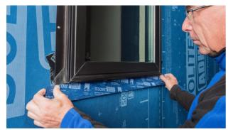
**18.1 Alternative: Sealing to flanged windows (USA)** Insert the window, fasten it and the seal with TESCON VANA on SOLITEX ADHERO all around the window in a waterproof manner. Rub tape firmly into place using the pro clima PRESSFIX application tool.
