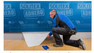
**10. Remove the remainder of the release film** Grip the wide release film by the previously folded corner and pull it off.
