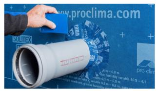
**23. Alternative with TESCON VANA** Alternatively, the pipe feed-through can be sealed in an interlocking pattern from top to bottom in a waterproof manner using TESCON VANA.
