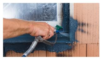
**8. Spray over AEROSANA FLEECE** The AEROSANA FLEECE is embedded in place by spraying again with AEROSANA VISCONN.
