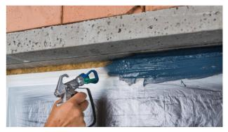
**4. Spray the lintel and reveals** Apply the required layer thickness of AEROSANA VISCONN in one or two spraying steps.
