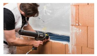
**6. Continue around the rest of the window** Bond all four sides of the frame to the masonry using AEROSANA VISCONN / FIBRE.
