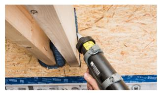
**5. Fill the joint** Fill the joint with a sufficient amount of AEROSANA VISCONN / FIBRE.
