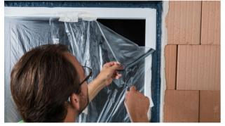
**9. Remove the protective sheeting** Remove the stuck-on protective sheeting before AEROSANA VISCONN dries.
