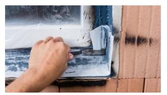
**7. Install the AEROSANA FLEECE sub-sill flashing** Insert the AEROSANA FLEECE into the still-wet AEROSANA VISCONN spray film, ensuring there are no folds or creases. Carefully finish any corners or raised edges.
