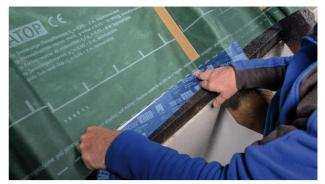
**5. Stick joints** Once the spray has dried, apply the adhesive tape and gradually stick it in place.
